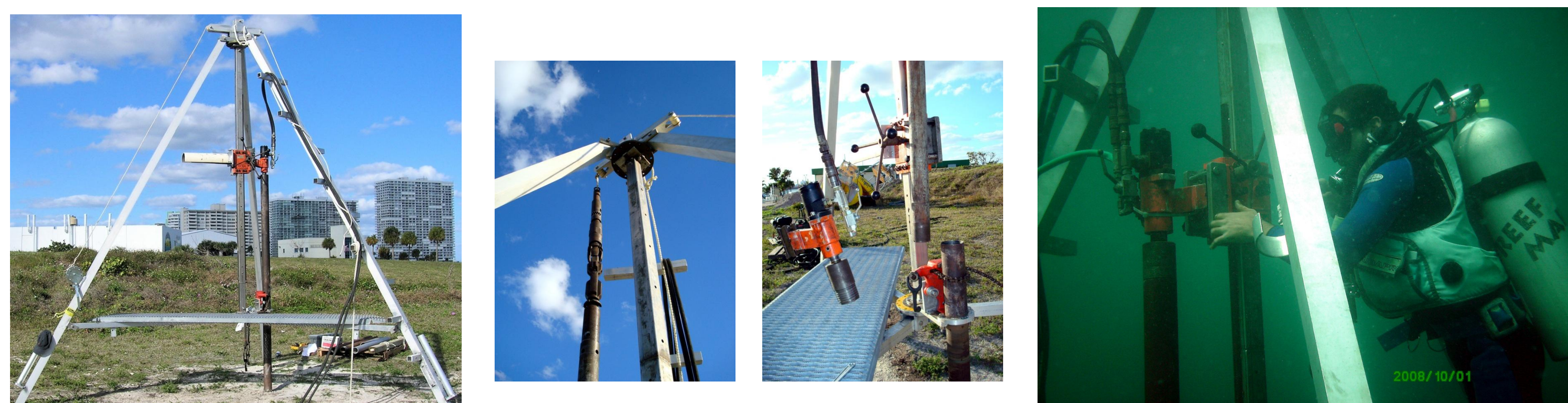
Figure 3: Images of tripod, drilling equipment, and underwater core-drilling
